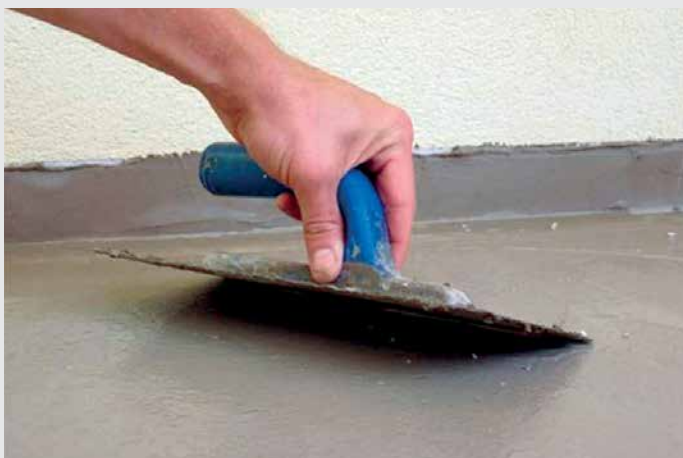
3. Aplicare Baumacol Baumit Protect
