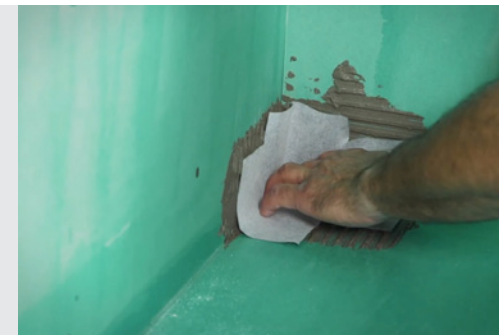
4. Fixare Baumacol InCorner Plus / ExCorner Plus / Sleeve / Gully
